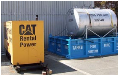
Figure 4-7 Picture of an external fuel tank connected
