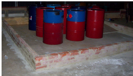
Figure 4-6 Bunded Fuel Storage Area
